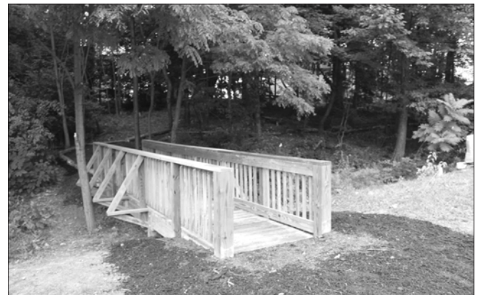
Finished pedestrian bridge at Boogersburg School.
