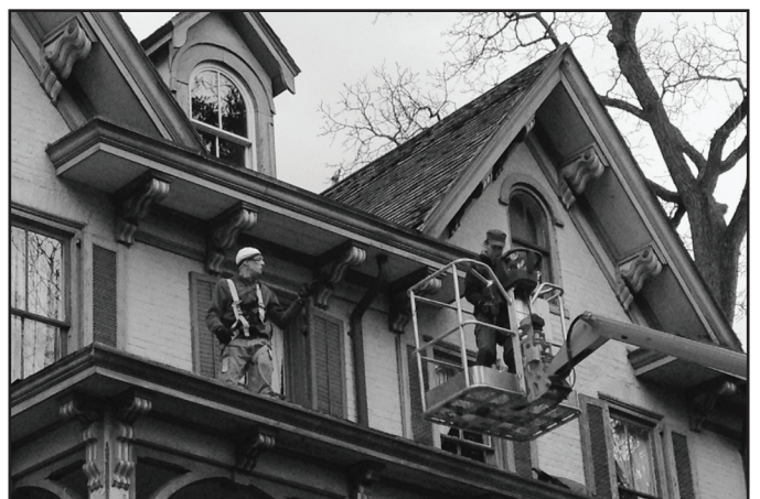
Two photos above: Nate & Maria Day of Sterling Stoneworks begin restoration of the Centre Furnace Mansion's front porch roof and balcony.
