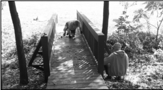
Rick Schutz, Ed DeBrasky and Paul Scanlon preparing the pedestrian bridge at Boogersburg School for painting on the Day of Caring.
