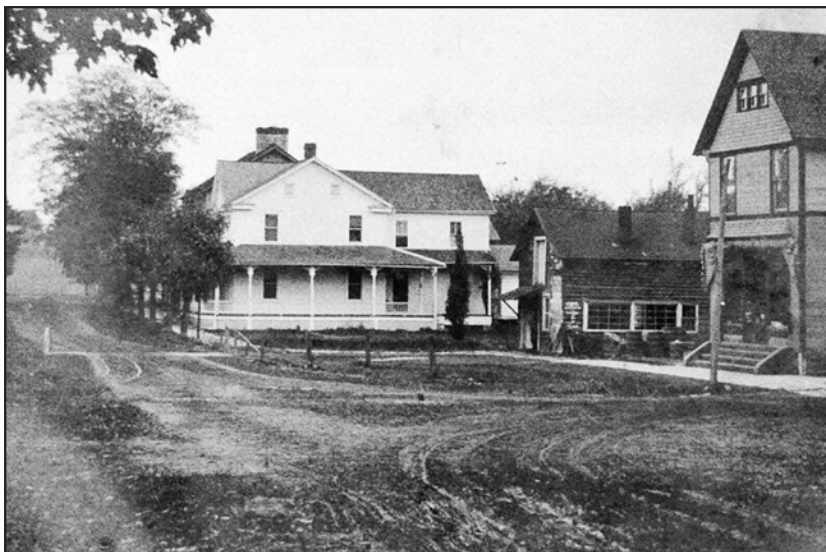
Main Street at the Diamond looking at former IOOF building, Boalsburg.
