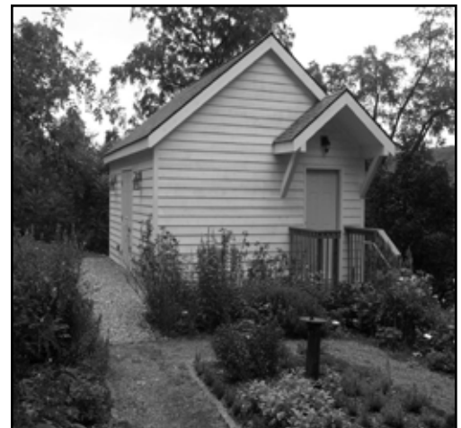
The completed Icehouse, overseen by Art Anderson
