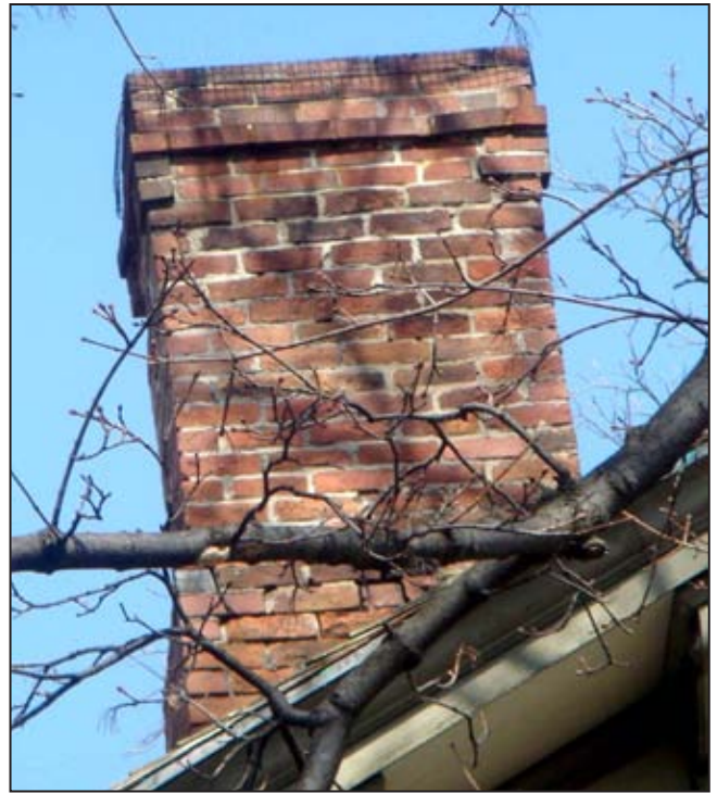
Northwest chimney before restoration.
