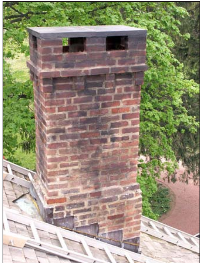
Northwest chimney after restoration.
