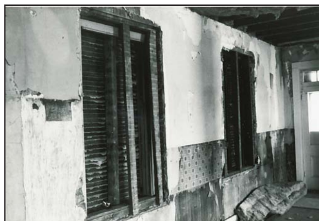
Removal of the “modern” kitchen from the current Library
