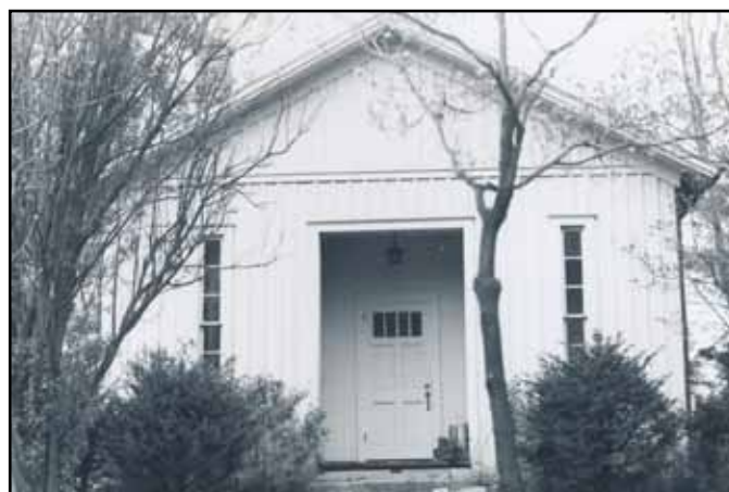
Boogersburg School: Historic Site Survey circa 1978-1981.
